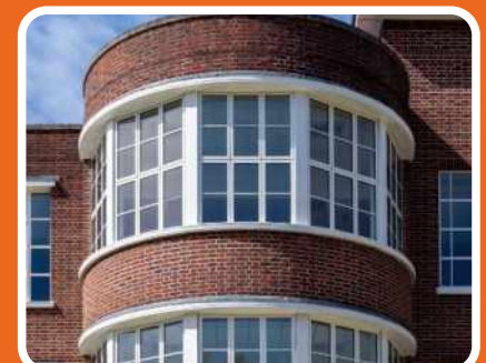
Meets Building Regs
